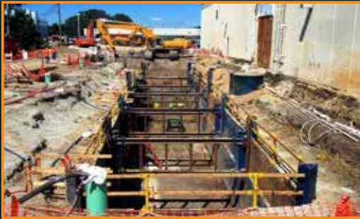
Slide Rail Shoring
