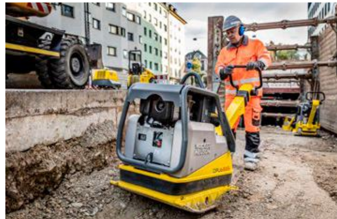
Safe in every case: If the guide handle is released, the unit only vibrates on the spot.
